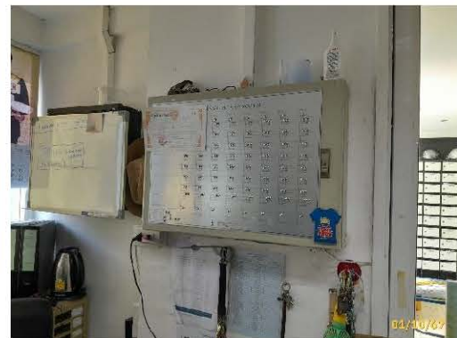
Fire Alarm Control Panel
